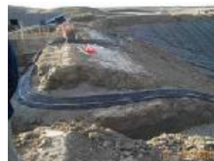
The biocell shell was constructed on one hectare of land at the City of Calgary's 240-hectare Shepard landfill site in 2004. It be... Full caption and actual photo size
