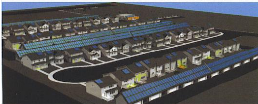
Above: computer generated view of the SAIC project subdivision combining solar energy panels with underground thermal energy storage.
